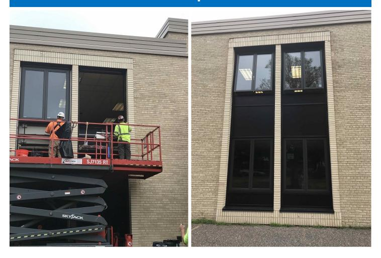
From left to right: Window removal underway; new windows and panels installed (June 2021)
